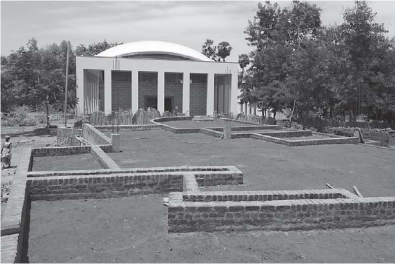
Phase 3 Construction, August 2005
